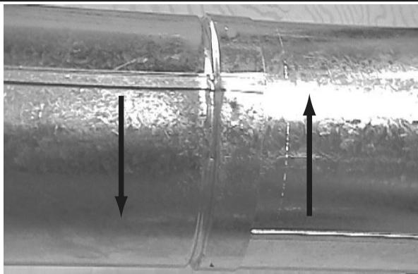
Figure 3.8 - Rotate Seams for Disassembly
