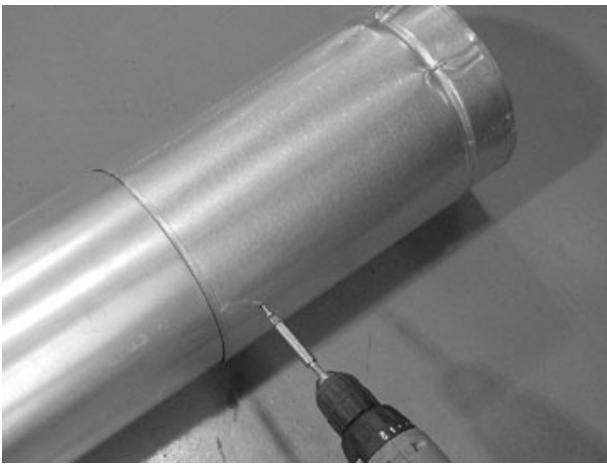
Figure 3.5 - Screws into Slip Section
