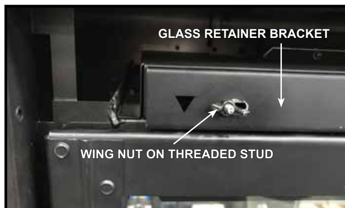
4.3 Glass Retainer Bracket & Wing Nut Detail
